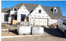
#1 – Dirt in street; Vegetative Buffer overrun by silt (1302 Oakhurst Cir.)
