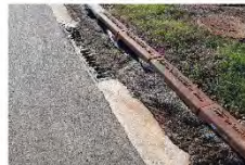
#11 – Flattened / degraded silt wattle
