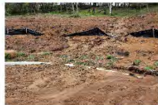
#1 – Downed silt fencing along Forest View Drive and sediment in the street (below white curb).
