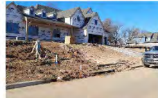
#2 – Dirt in street; No Silt Fence; No Drain Protection (2787 Forest View Drive)
