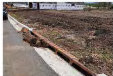
#4 – Partially unprotected storm drains on west end of Pinecrest Dr.
