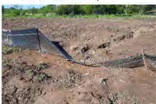
#5 – Overwhelmed silt fence near dead end of Forest Hill Way
