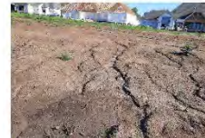
#12 – Example of rill erosion observed along Cedarwood Drive leading to soil in roadway at Forest Hill Way
