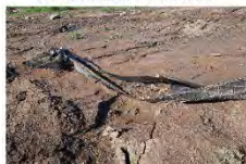
#6 – Overwhelmed silt fence near dead end of Forest Hill Way
