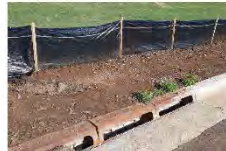
#9 – Partially unprotected storm drain along Forest View Drive
