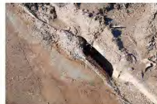
#7 – Partially unprotected storm drain at dead end of Forest Hill Way
