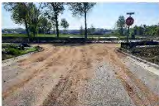
#1 – View of sediment on Forest Hill Way spilling onto Cedarwood Drive
